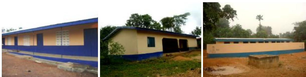
Otaipro 3-unit Primary School block Ofoase Kuma 3-unit KG Classroom block Kwahu Nsaba 10-seater KVIP Toilet
