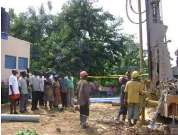
Drilling of Boreholes at the Epicenters
